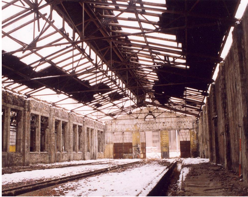
Figure 4. The pre-restoration state of Hangar 1-2 (Uygur Architecture Archive, 2019)
