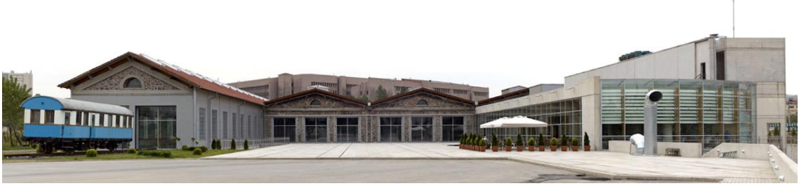
Figure 1. Post-restoration view of CerModern from the courtyard (Cemal Emden, 2010)
