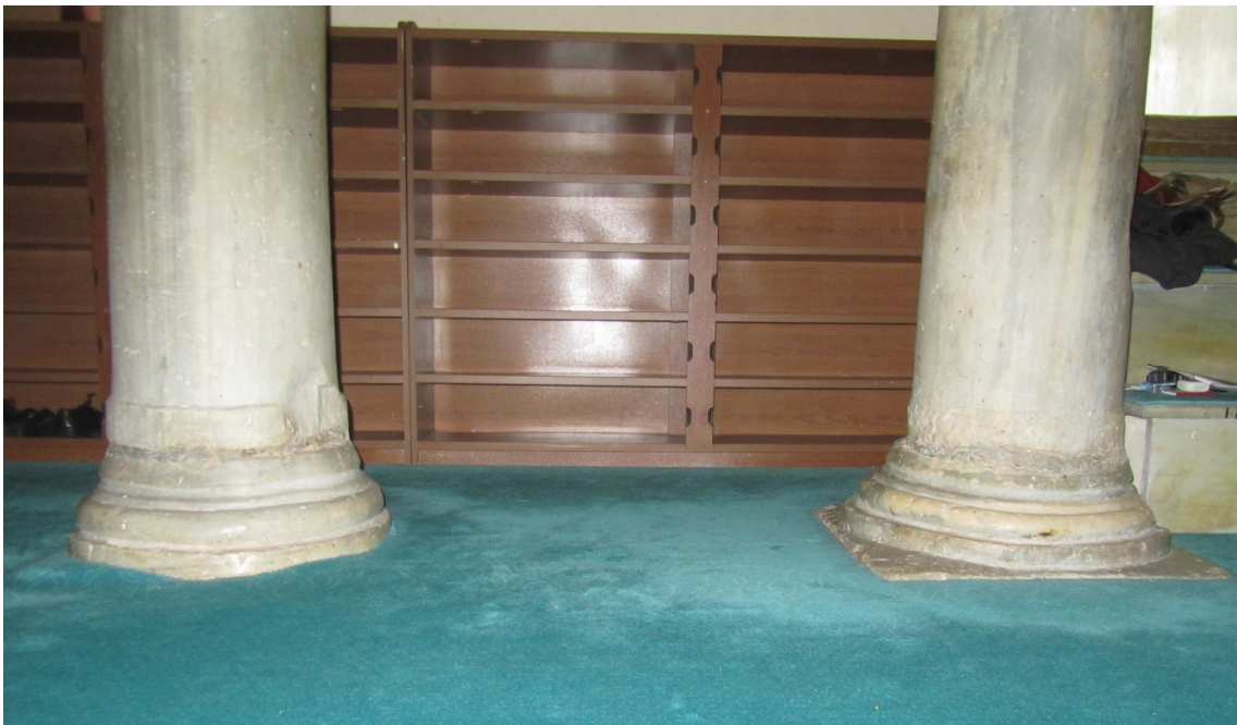
Fig.7. Attic-type column bases
