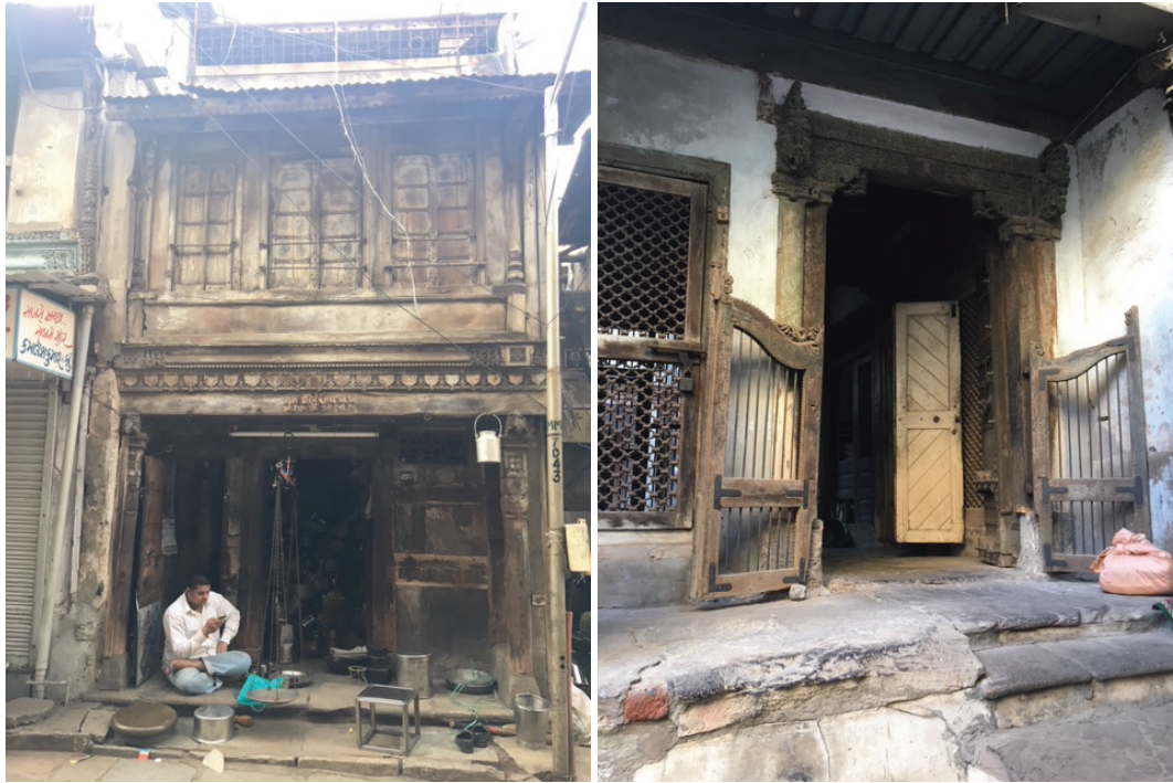
Figure 4 and 5: Typical facades of pol houses
