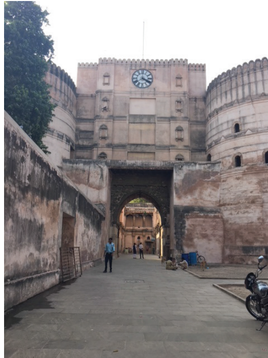
Figure 2. The Bhadra Citadel
