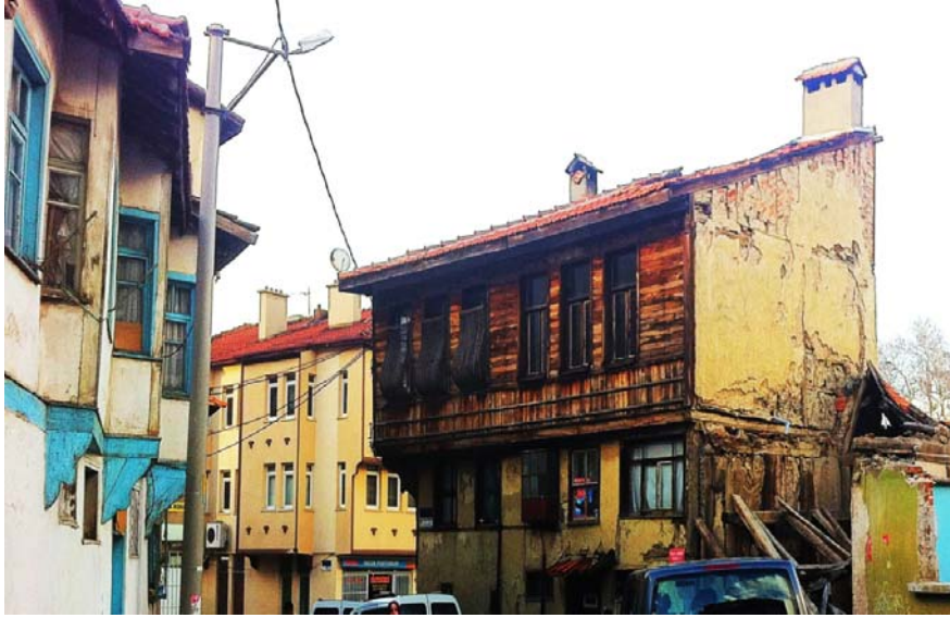
Figure 2. Buttress and outbuildings wooden houses (writer archive,2014)
